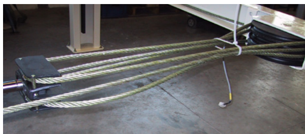
Figure 4.23 Securing the cables to the piston head
