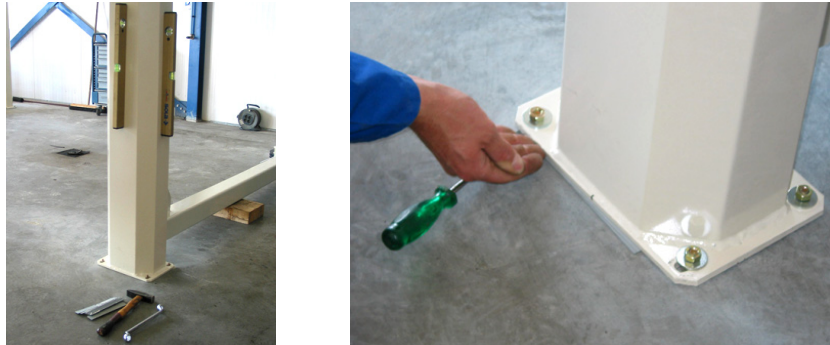
Figure 4.9 Vertical positioning of the posts
