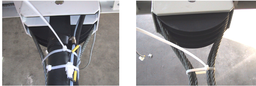
Figure 4.26 Binding the cables together
