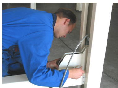
Figure 4.18 Assembly of cable pulleys
