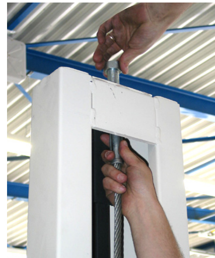
Figure 4.20 Cable run crossbeam I - II and in the posts
